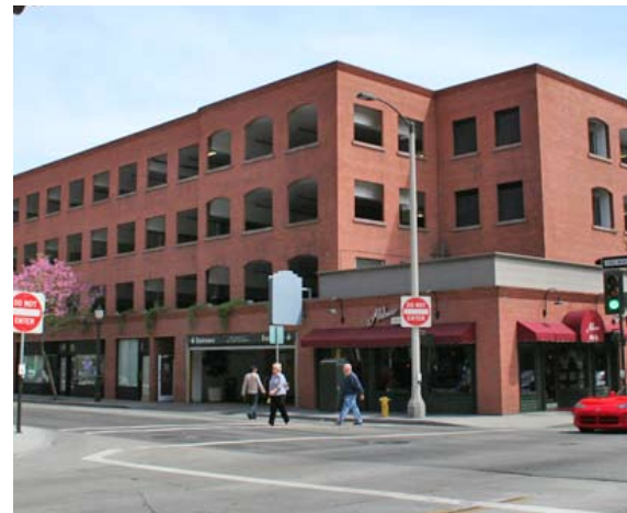
Parking garages may be phased in over time as an area develops. Mixed-use parking garages with retail on the ground floor blend in well with their surroundings.
