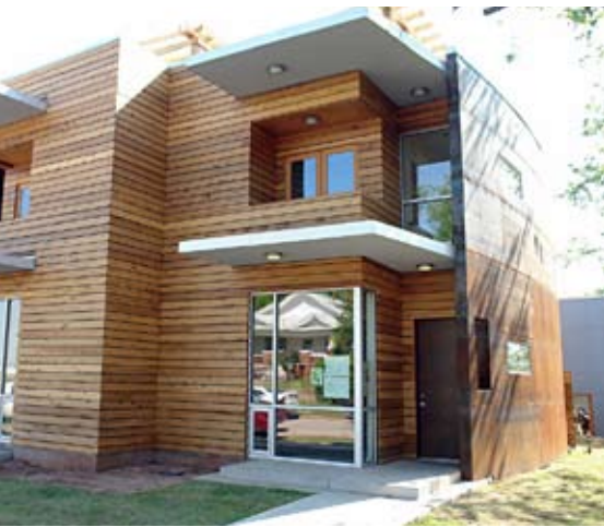
U.S. Green Building Council
